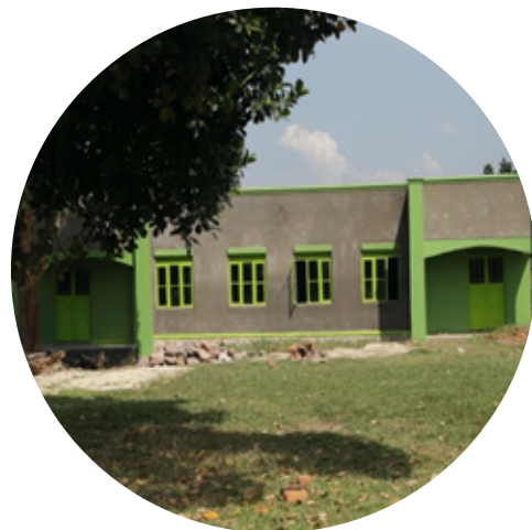
The new classroom block built by the Motara family.
